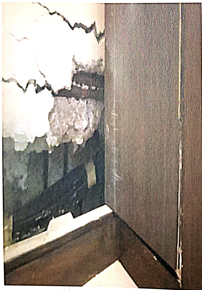
MAJOR COLUMN DAMAGED HAS BEEN OBSERVED INSIDE FLAT
