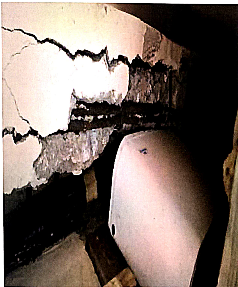
MAJOR COLUMN DAMAGED HAS BEEN OBSERVED INSIDE FLAT
