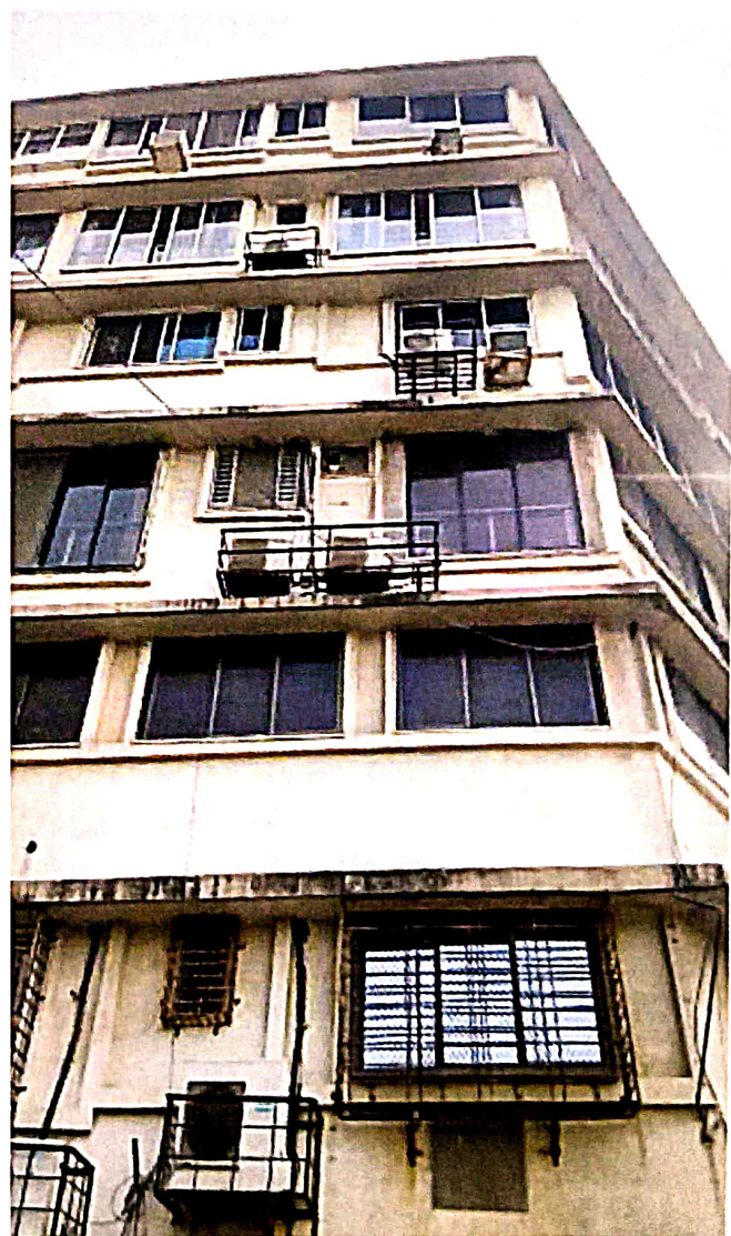
Noticed Chajja found highly damaged condition
