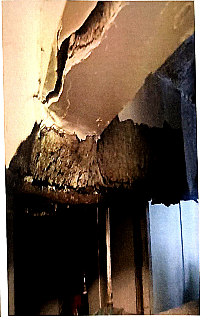
MAJOR COLUMN DAMAGED HAS BEEN OBSERVED INSIDE THE FLAT
