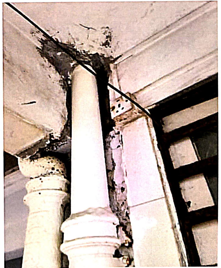
NOTICED LEAKAGES NEAR PIPES AND PLASTER DAMAGE
