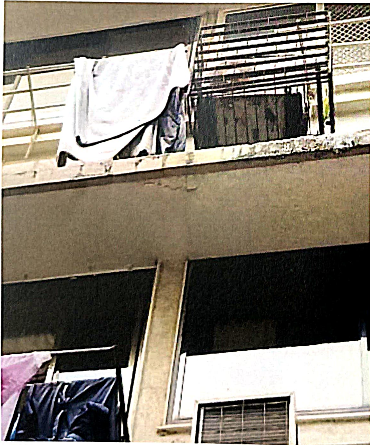
Noticed plaster damages at External wall of the building
