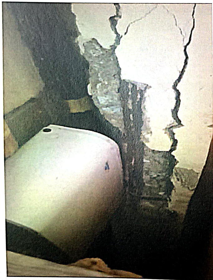
MAJOR COLUMN DAMAGED HAS BEEN OBSERVED AT INSIDE FLAT
