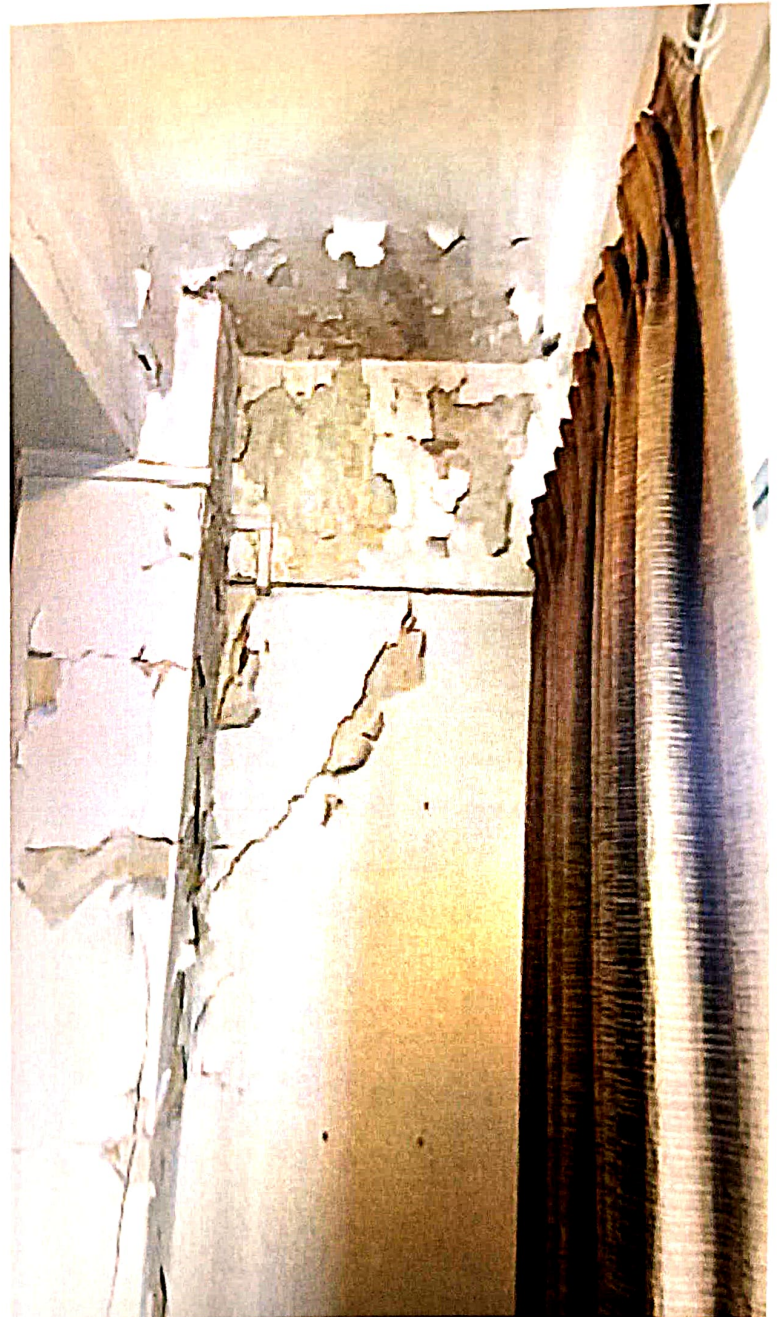
NOTICED LEAKAGE IN CEILING AT BEDROOM AREA
