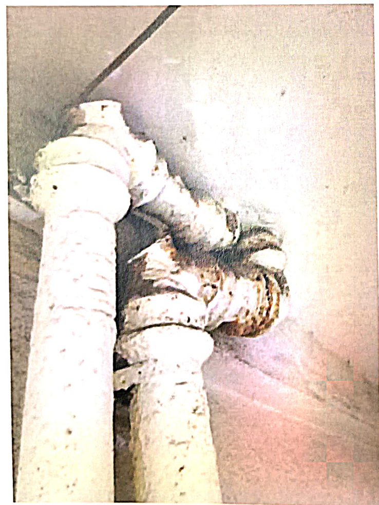
NOTICED LEAKAGES NEAR PIPES AND PLASTER DAMAGE
