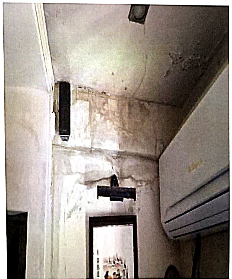
NOTICED BEDROOM CEILING LEAKAGE
