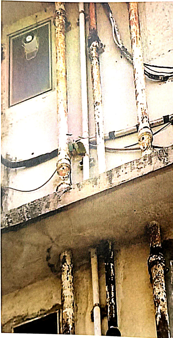
NOTICED MAJOR LEAKAGES NEAR DRAINAGE PIPES.
