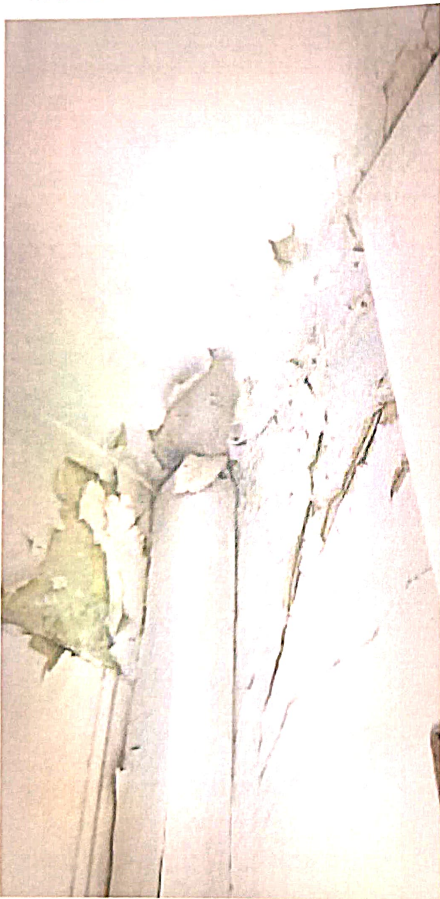
NOTICED LEAKAGE IN CEILING AT BEDROOM AREA
