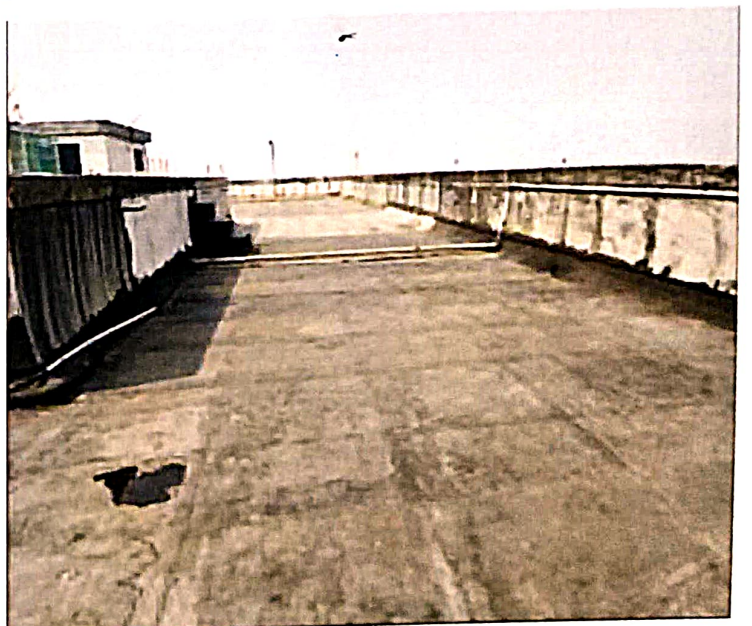
TERRACE FLOOR AREA DEVELOPED AIR POCKETS AT MANY PLACES
