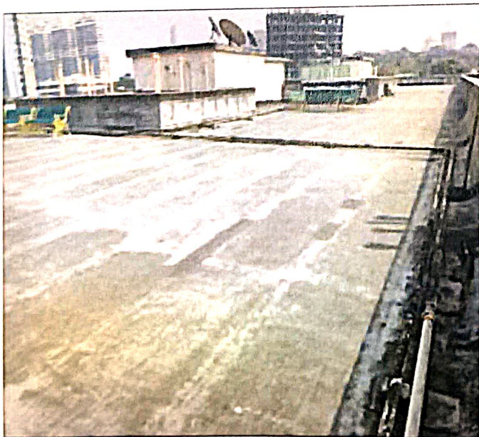
TERRACE FLOOR AREA DEVELOPED AIR POCKETS AT MANY PLACES
