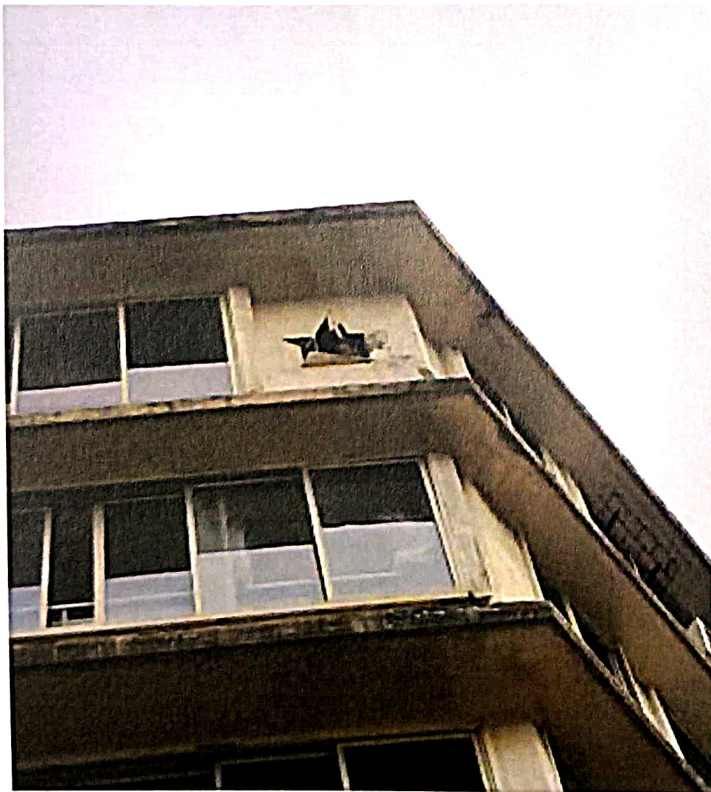
Noticed plaster damages at External wall of the building
